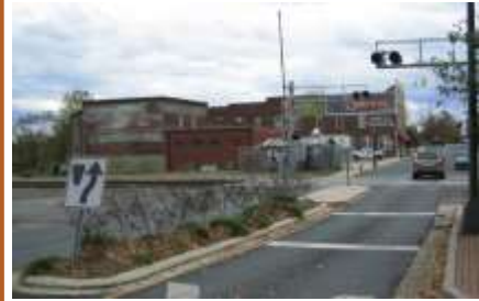
A median separation for the Rolla Street railroad crossing would make the crossing safer and could help to eventually make Rolla a “Quiet Zone”. A Quiet Zone would lift the requirement for passing trains to sound their horns. This noise can be a disturbance to surrounding residential areas.
